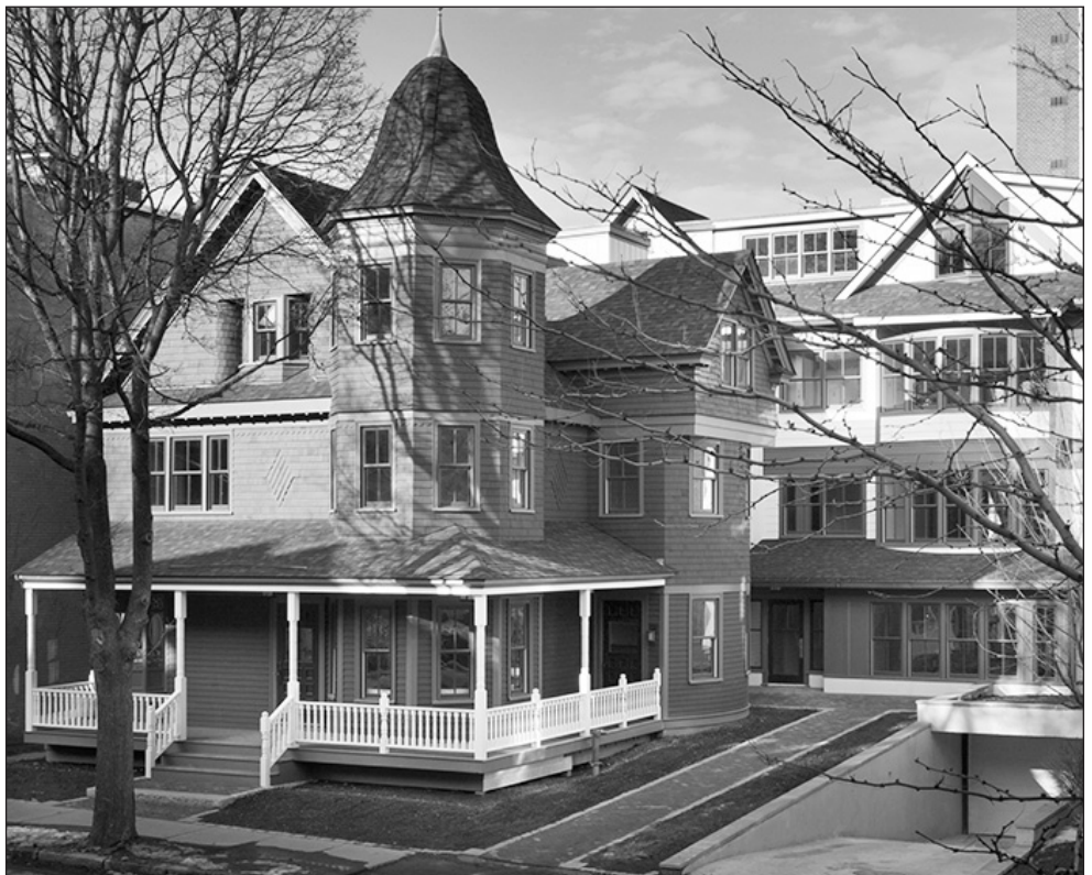
A five-unit luxury residential property at 99 Winchester St. will be the first LEED-certified condominium development in Brookline, Mass.
