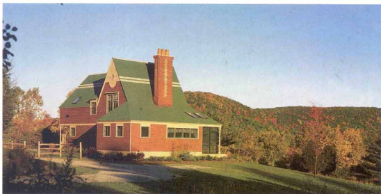
Colors inspired by the hills. The steep roof, the green shingles and the brown siding of this home were suggested by and designed to blend with the rolling Connecticut hills that surround it. Photo taken from B on floor plan.
